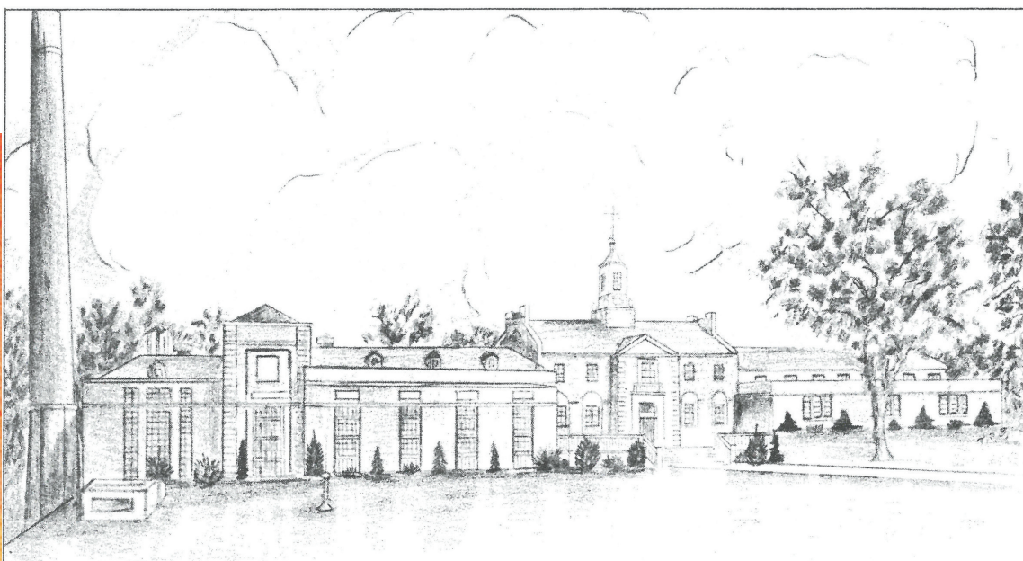
SPRINGFIELD CITY WATER COMPANY PUMPING and PURIFICATION PLANT
