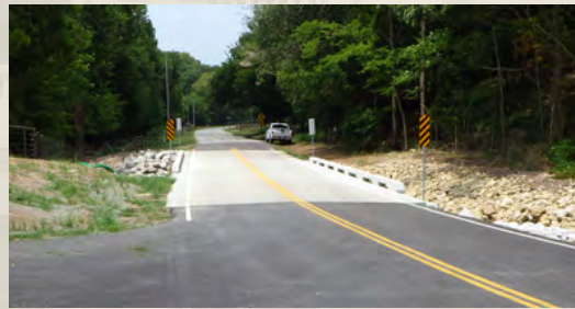
FARM ROAD 117 BRIDGE (OVER BRANCH OF LITTLE SAC)
