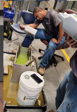
Luke & Nate cleaning the heat strips in the humidifier at Building Ops.
