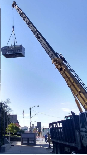
Lifting RTU 10 up on the roof of the old jail in 2020.
