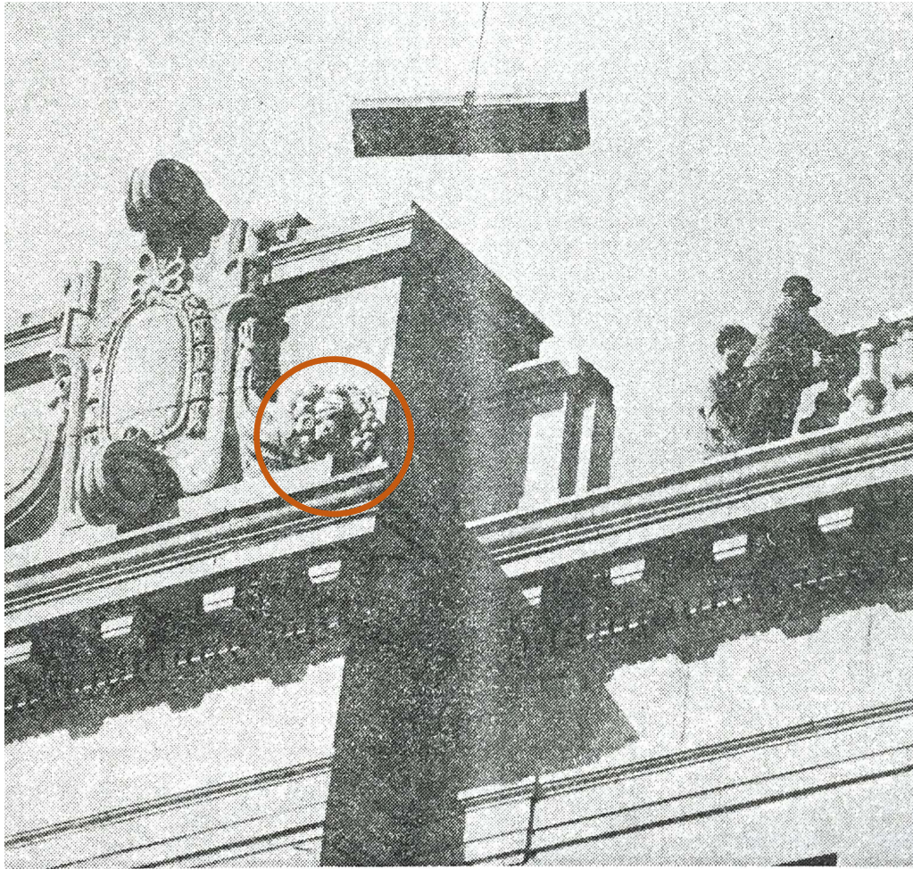
Parapet Removal – 1973 – Photo by Betty Love
