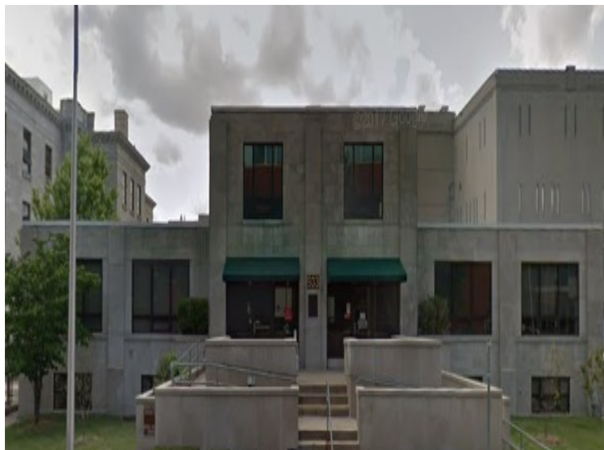
933 N Robberson Facility
