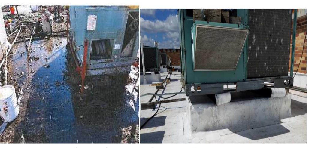
Wet insulation due to condensation from HVAC units Prevention: Units were raised and plywood placed over the curbs and covered with TPO
