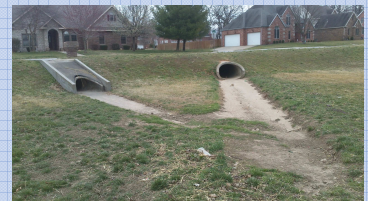
Figure 16: Outfall screening location
