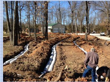
Figure 14: Lateral Line Installation Inspection
