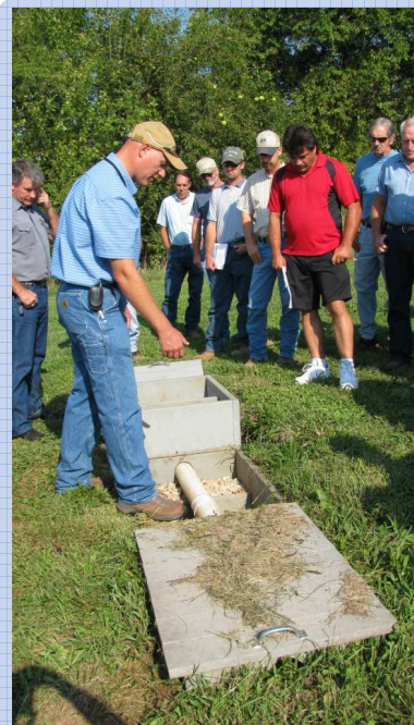
Figure 10: Greene County inspector Michael Bowers demonstrates a shallow-placement lateral line during a training for OSW installers and designers at the training center at Valley Water Mill
