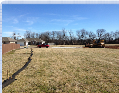
Figure 17: Construction Site BMPs
