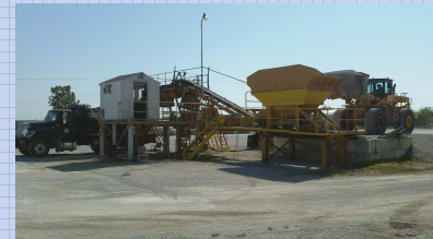
Figure 23: Cold mixing asphalt
