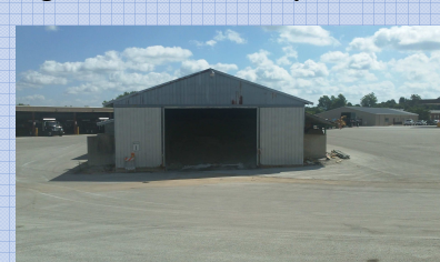
Figure 26: Clifton Facility salt storage barn
